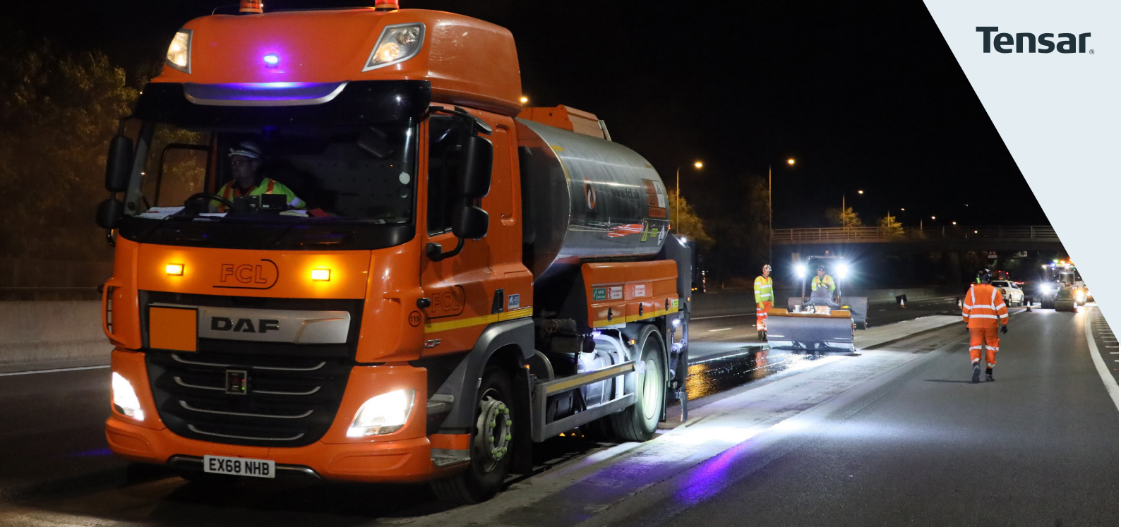
Installation of Tensar Glasstex P100
