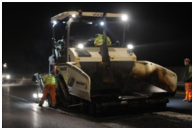
Due to the instant break time of the 160/220 pen bitumen bond coat, Toppesfield could proceed rapidly with installation of the final 75mm AC 14 EME binder and the surface course system.
