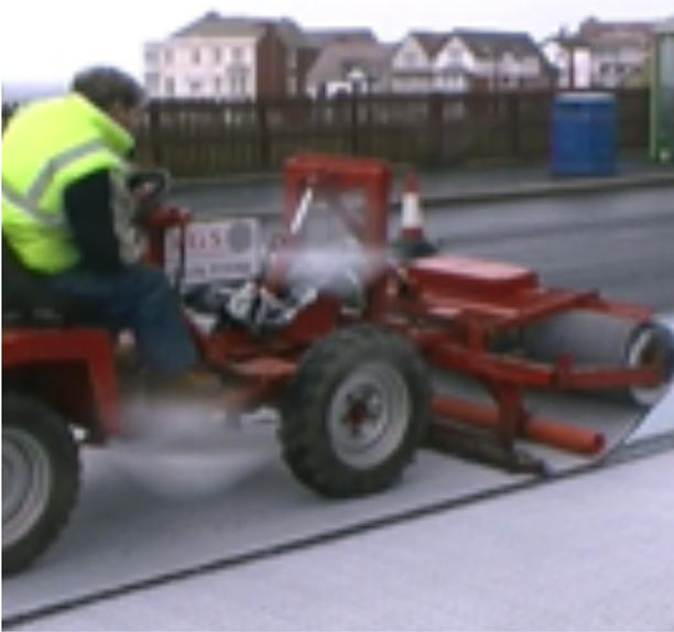
The existing asphalt was milled off to a depth of 50mm and a pre-regulated asphalt surface 25mm thick was placed. 200 pen bitumen spray was then applied and 11,000 m<sup>2</sup> of Glasstex® P100 was installed using a purpose built lay-down machine for speed and accuracy by specialist installer AGS Ltd, now operating as Foster Contracting Ltd. A 14mm stone mastic asphalt (SMA), 40mm thick surfacing course was then placed directly on to the Glasstex®.
