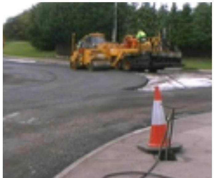
A conventional HRA base course followed by a 30mm thick asphalt surfacing layer was machine laid directly over the Glasstex® on the roundabout and on to a tack-coated milled surface on the adjoining A505. In 2005 this resurfaced but unreinforced adjoining A505 had deteriorated to a degree that the client decided to resurface it, while the roundabout was deemed not to warrant re-surfacing.
