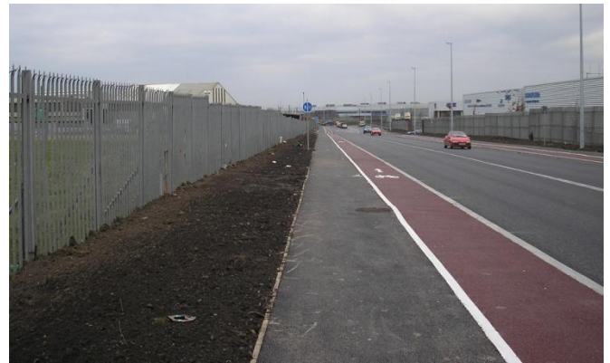
Road after upgrade
