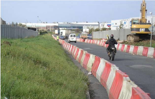
Road before upgrade
