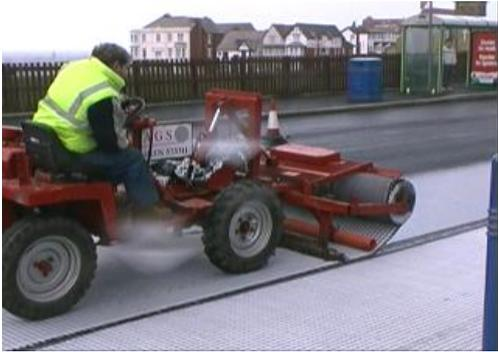
Glasstex<sup>®</sup> is rapidly machine installed
