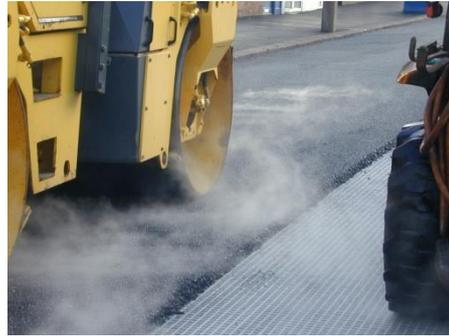
Surfacing is placed directly on Glasstex<sup>®</sup>
