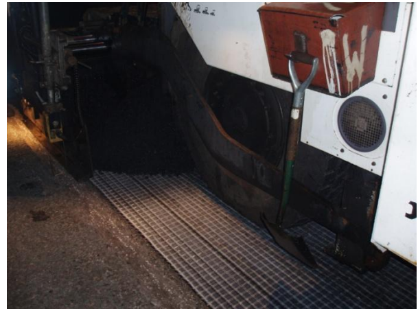
Binder course placed directly onto Glasstex
