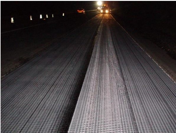
Glasstex is bonded onto the planed surface
