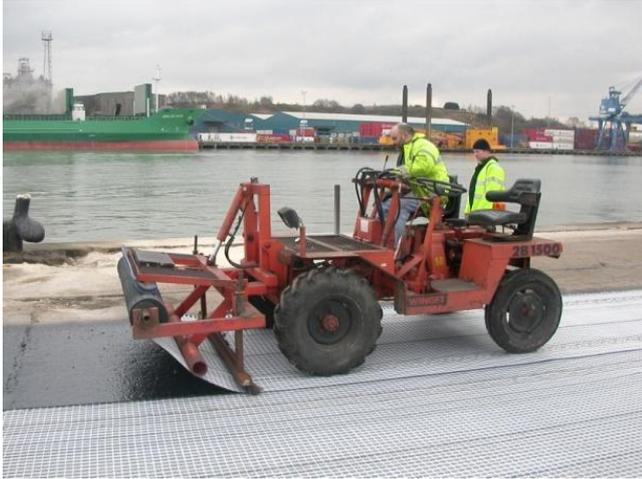
As soon as the Glasstex had been laid it was ready for placement of the 55/10 hot rolled asphalt (HRA) surfacing. This was laid in a single 45mm thick layer using a conventional paver.
