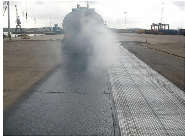
Fosters then machine installed the Glasstex P100, using their specially developed Geosynthetic Applicator.
