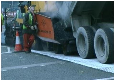
Paving directly on to the Glasstex
