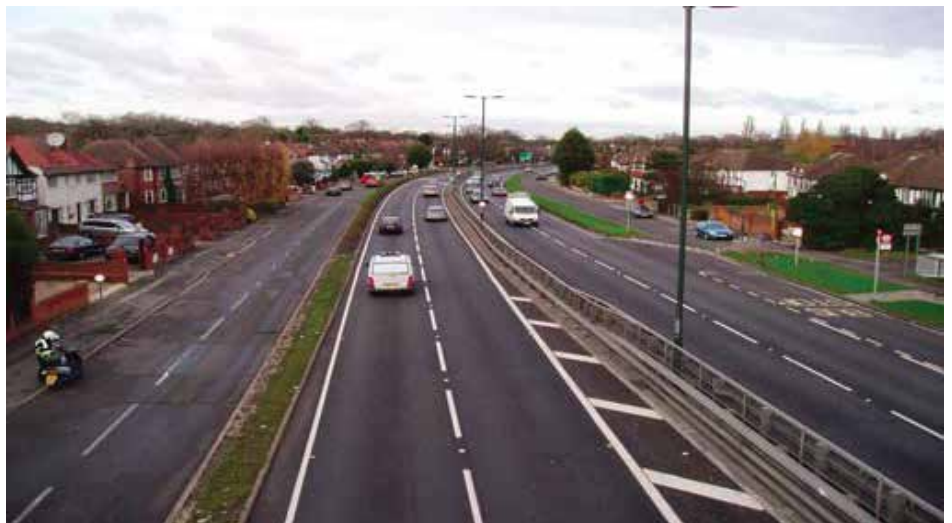
The restored carriageway
