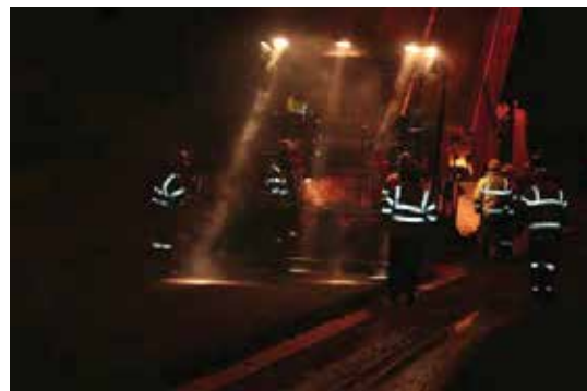
Installation of the wearing course
