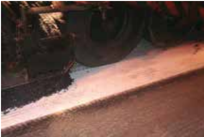
Installation of the wearing course
