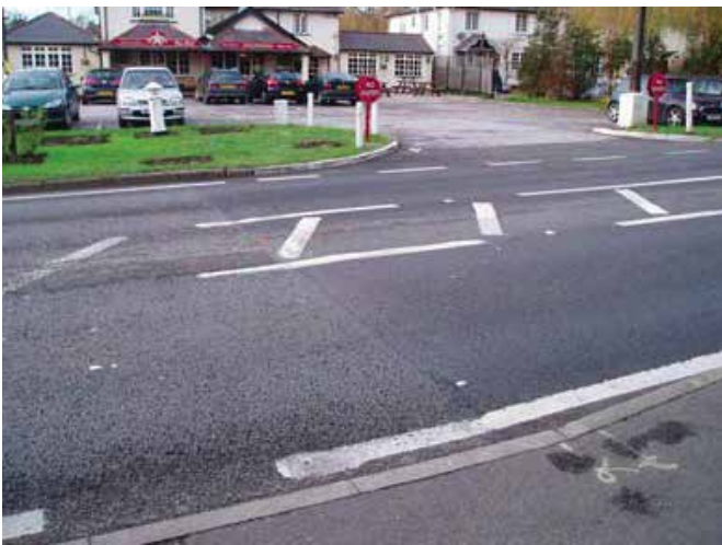
Join in the surface showing start of the project
