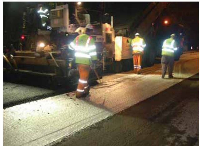
Installation of the 200kN/m geosynthetic
