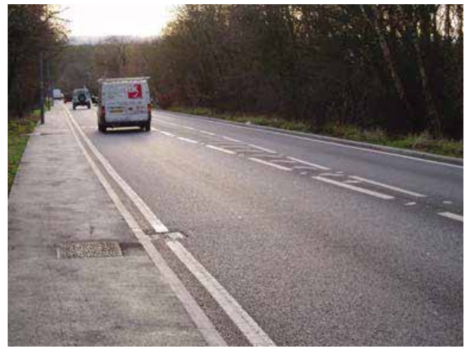
The refurbished carriageway
