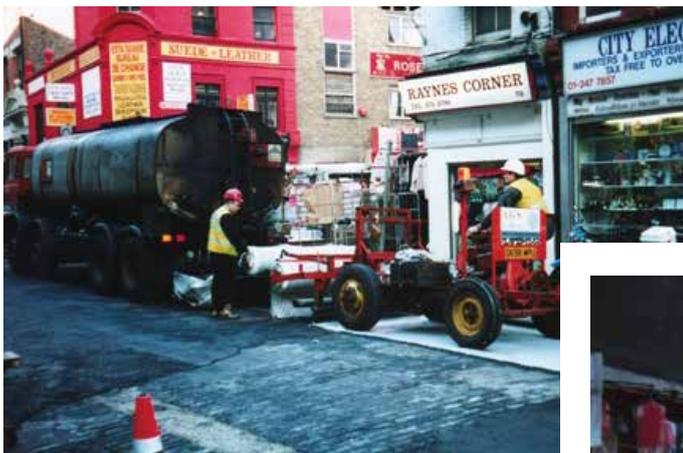
*Installation of the 100kN/m composite*
