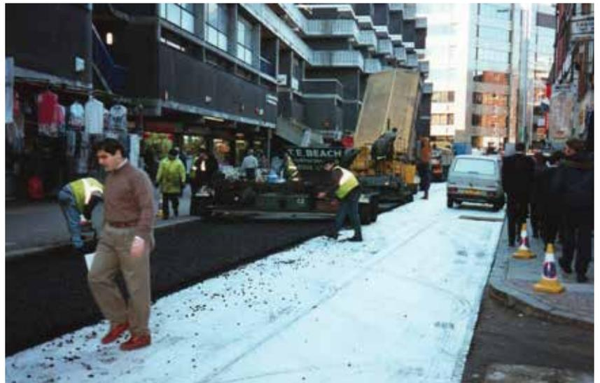
*Hot rolled asphalt surfacing*
