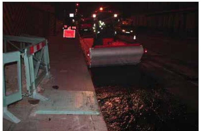
*Installing the composite onto the bond coat*
